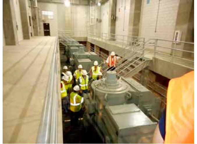
YPs learning more about the concrete volute pumps from Mr. Shane Keil (Smith Pump Co.) and Mr. Ed Smith, P.E. (Jacobs).
