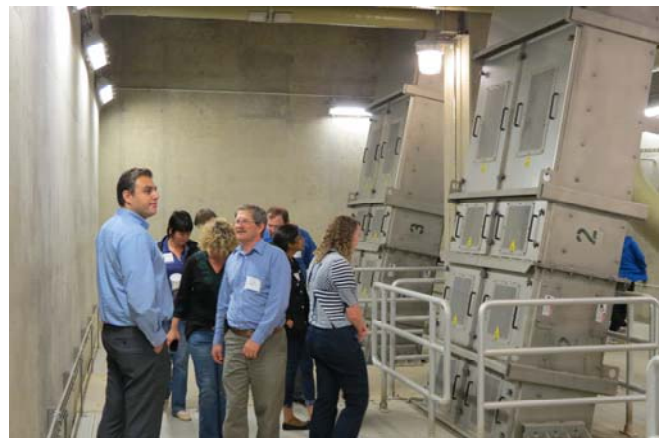
IPS Tour in Progress. Screening mezzanine level pictured.
